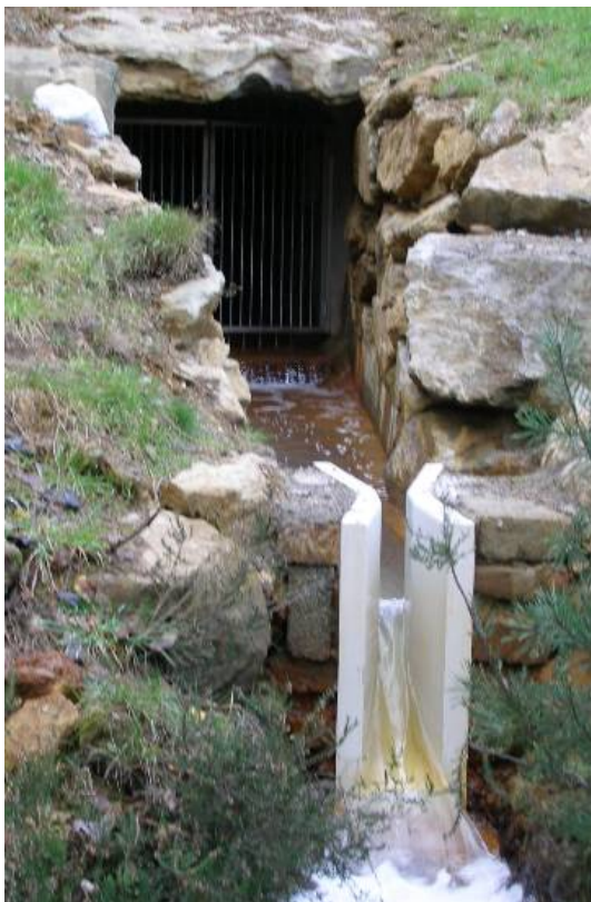
Above: Road Adit, West Avoca, Co. Wicklow
