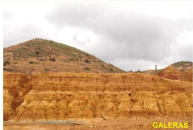
**Fig. 2** Barren and severely eroded slopes of the studied tailings impoundments, showing a high density of rills and gullies
